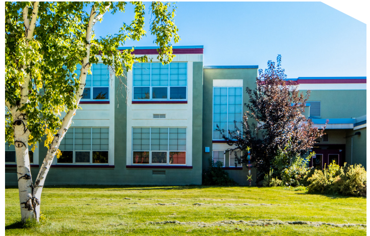
Hawthorn Elementary School Bozeman, MT
