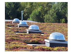
Description: This session will study inspiring applications of Tubular Daylighting Devices (TDDs) around the world that deliver natural light into unique spaces and create visually appealing natural lighting to complement an overall design.
