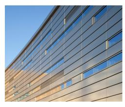
Description: Maximizing Envelope Performance with IMP-Integrated Components explores an advanced insulated metal composite panel building envelope system, components that have been engineered to integrate with the system - including windows, daylighting panels, sunshades, and louvers - and how the IMP system and integrated components combine to create a high-performance building envelope.
