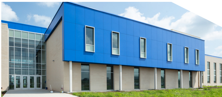
Junction City High School / Junction City, KS Swisspearl
