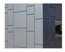
**Description:** As part of a well-designed rainscreen system, single-skin metal panels offer unique aesthetic options combined with the assurance that the building envelope will withstand the effects of long-term exposure to the elements. This course compares common cladding types; presents single-skin metal panel materials, coatings, finishes, and design options; and examines using single-skin metal panels with a single-component barrier wall to form a complete rainscreen assembly.
