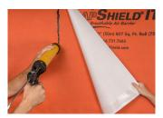
Overlap vertical seams by min. 12". Apply ¼" (6.4 mm) bead of VaproBond adhesive sealant to ensure water and air barrier seal.
