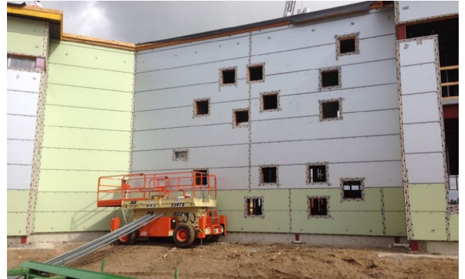
2. Genwall panels are extremely versatile and allow for windows to be cut anywhere.
