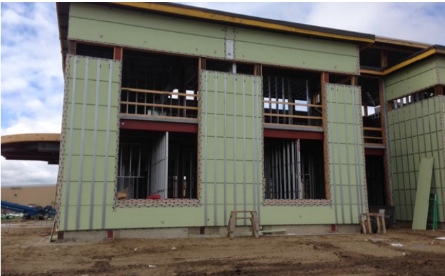
3. Genwall panels maximize the length of the space along the south elevation.
