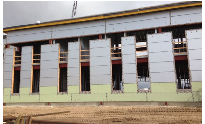
4. Genwall panel cuts can be reused in between spaces for cost effectiveness.
