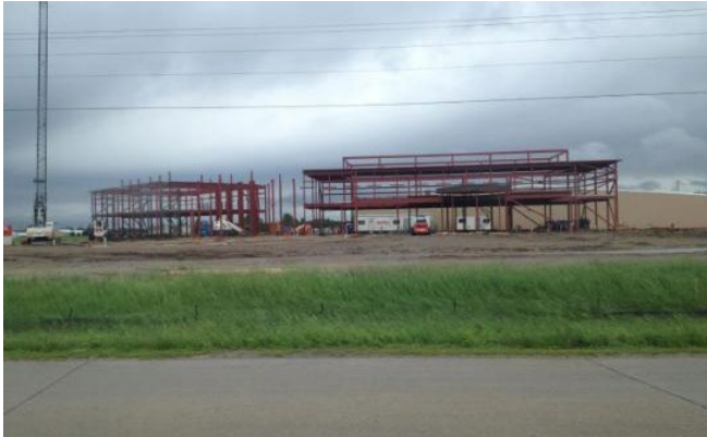
1. Construction begins on Sukup Manufacturing Co.
