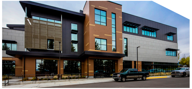
Helena Readiness Center / Helena, MT Kalwall / Solatube
