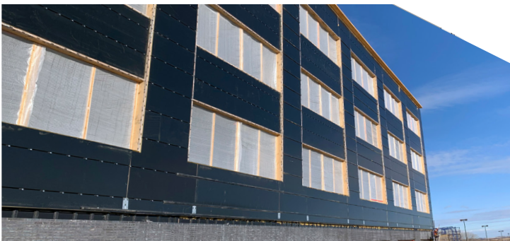
SCC Health & Sciences Building / Lincoln, NE Genwall Insulated Backup Wall System
