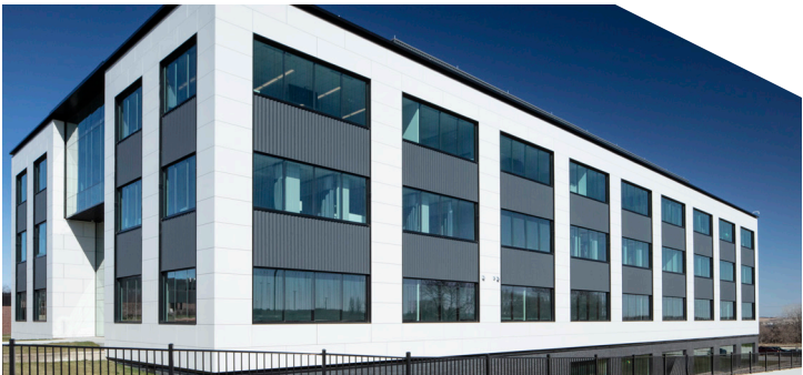
SCC Health & Sciences Building | Lincoln, NE Genwall & Swisspearl
