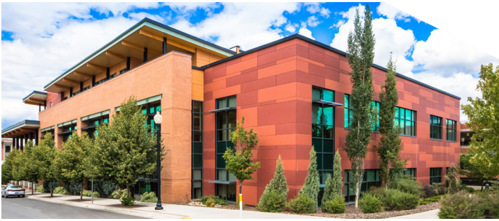
Montana State Fund Bank / Helena, MT Swisspearl, Kalwall, & Misc.
