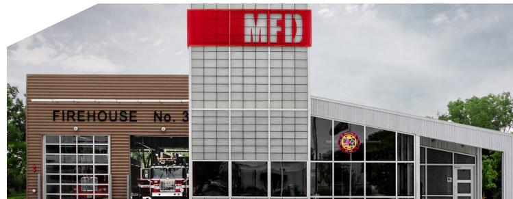
Manhattan Fire Station No. 3 - Manhattan, KS / Kalwall
