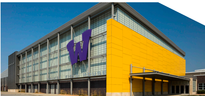
Waukee High School / Waukee, IA Centria & Kalwall
