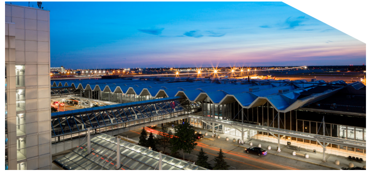
Minneapolis International Airport / Minneapolis, MN Centria & Sieccoline
