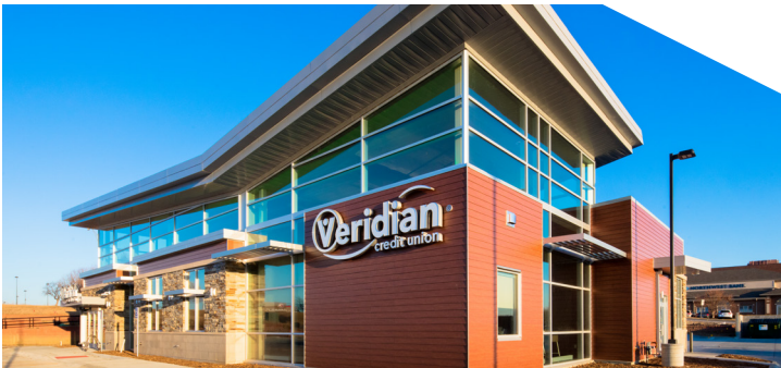
Veridian Credit Union / Council Bluffs, IA (4 Omaha-metro locations) Genwall, Siecoline (ACM), & Phenolic Panels
